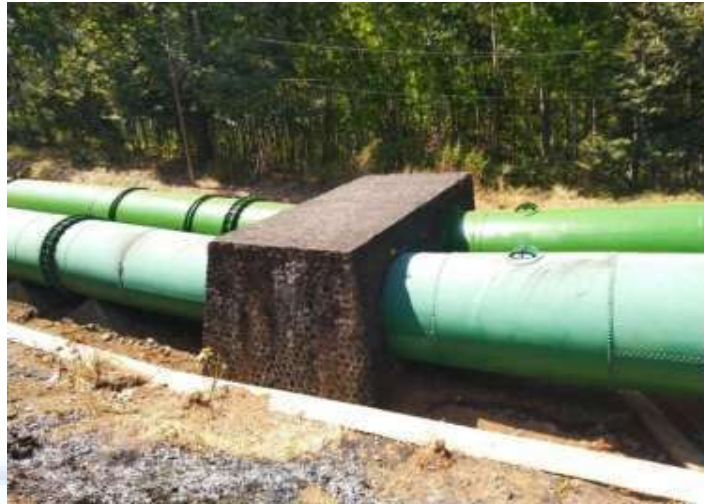
Gambar 2.5 Pipa pesat ( Penstock )
